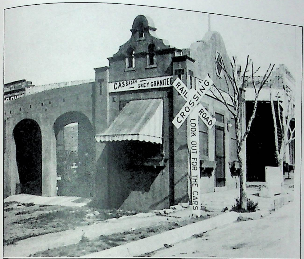
This was the Cassaday Grey Granite Co. – Chrissy's Bakery is now located in this building. The building was built in 1910 by Cassaday, and his company was the first to use motor transportation for hauling granite.
